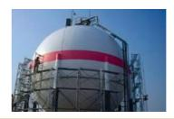
Gas Tank - China Solacoat Metal Roof System applied to gas tank in China to reduce heat built up to lessen gas losses.
